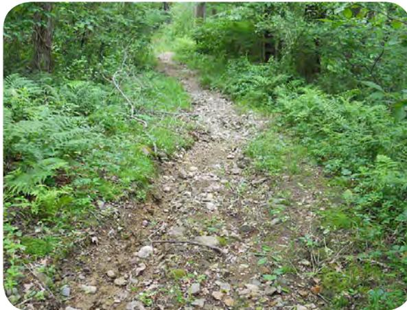
*Surface* is uneven, with signs of wear and minor erosion on unpaved trails and cracks or damage on paved trails. *Signage* has damage or graffiti that affects its legibility. Poles are leaning or are unstable. *Drainage* issues cause some trail erosion during rain; muddy areas or pooled water appear after a rain, but use is only occasionally affected.
