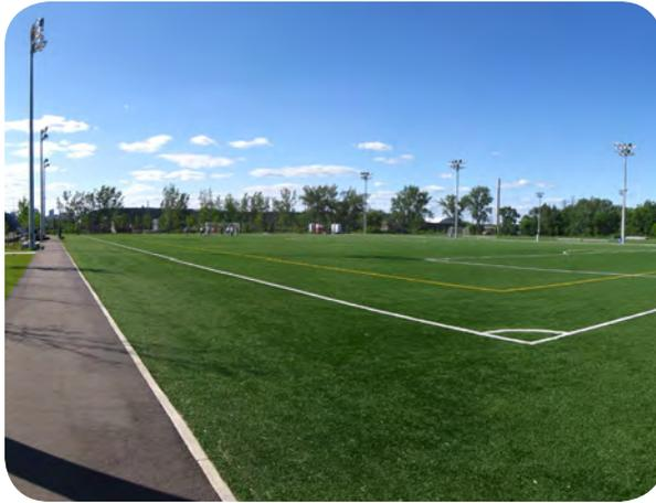
*Field Surface* is flat and obstacle-free, turf and infill density is consistent across the field. Permanent markings are fully intact and legible; *Irrigation System* applies water evenly and efficiently. All heads, valves and controllers are in proper working order; any leaks are minor and infrequent; *Drainage* is functional, water does not pool or flow at excessive rates; *Lighting Fixtures (if present)* are in good repair and allow evening play.
