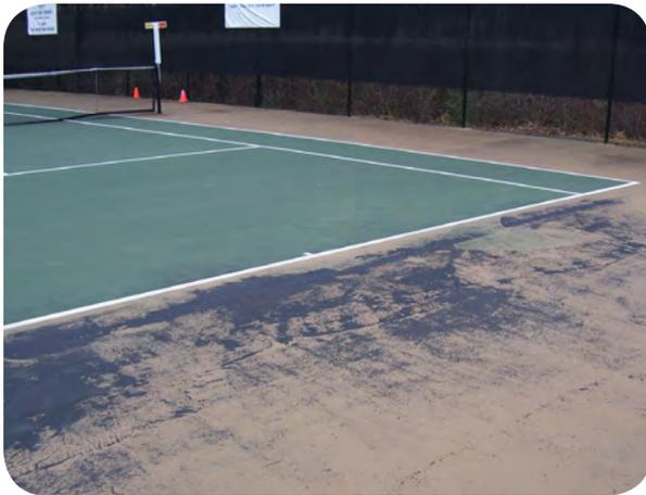
*Playing Surface* is playable but has some cracks, a slightly uneven surface, or paint that is chipped and worn. Net supports may be leaning but still hold up the net; *Drainage* issues leave the court susceptible to pooling of water that occasionally limits play; *Lighting Fixtures (if present)*: need some repair or replacement; evening play is possible but uneven lighting affects play; *Enclosure (if present)* is damaged in some sections, resulting in the occasional loss of tennis balls.
