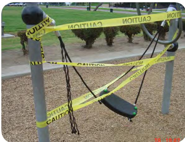
*Play Equipment* needs major repairs or replacement to be compliant with safety standards. Damaged or missing components limit play opportunities. *Safety Surfacing* is absent or damaged beyond repair in multiple areas. Loose material is not contained and requires frequent replenishment. *Drainage* is poor and regularly affects use. Rain and/or irrigation create large areas of pooled water or mud that limit use and damage safety surfacing.
