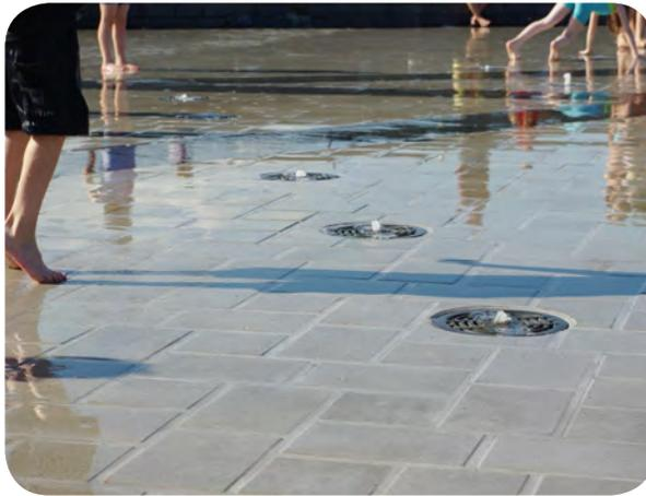
*Plumbing/Drainage* needs repair on average once a month; minor drainage issues result in pooled water when splash pad is off. *Nozzles/Spouts* are mostly operational; damaged equipment does not impact use. *Surface* of splash pad has minor cracks or chips that need repair, but still meets safety requirements.
